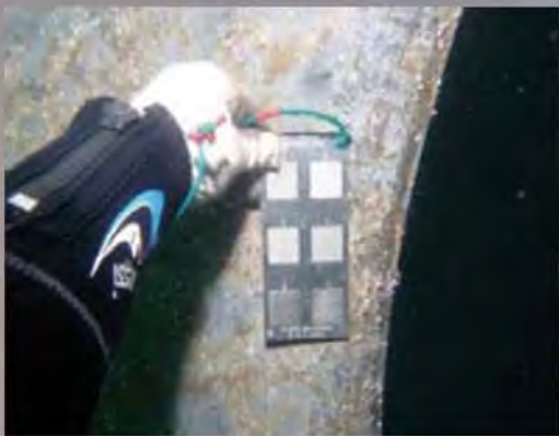
After Cleaning Condition
